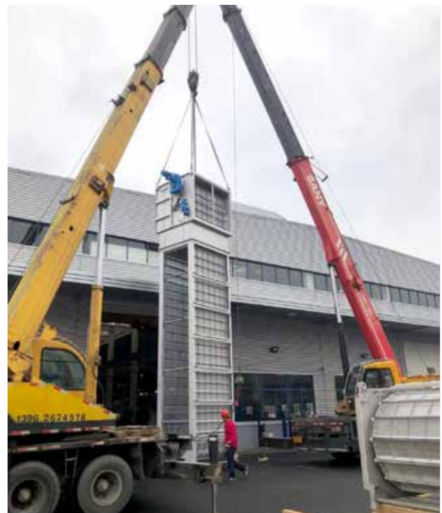
Delivery and installation of a HUBER Belt Screen CenterMax®.
